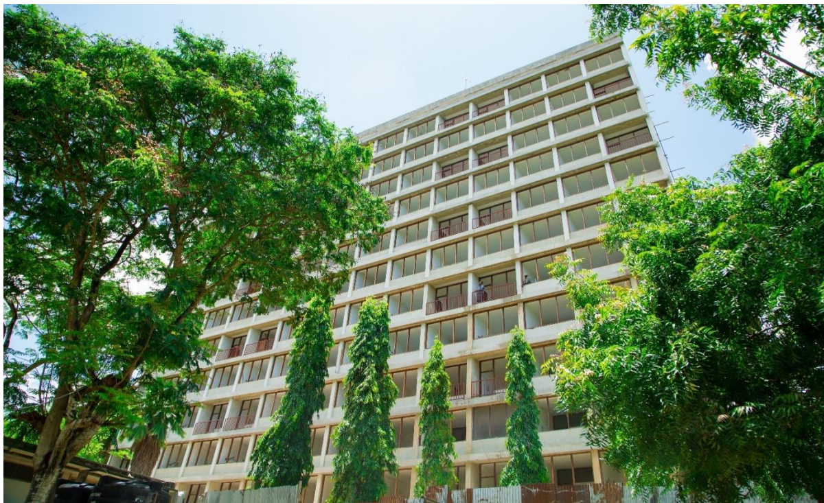
Rehabilitation of Students' Halls of Residence in Progress
